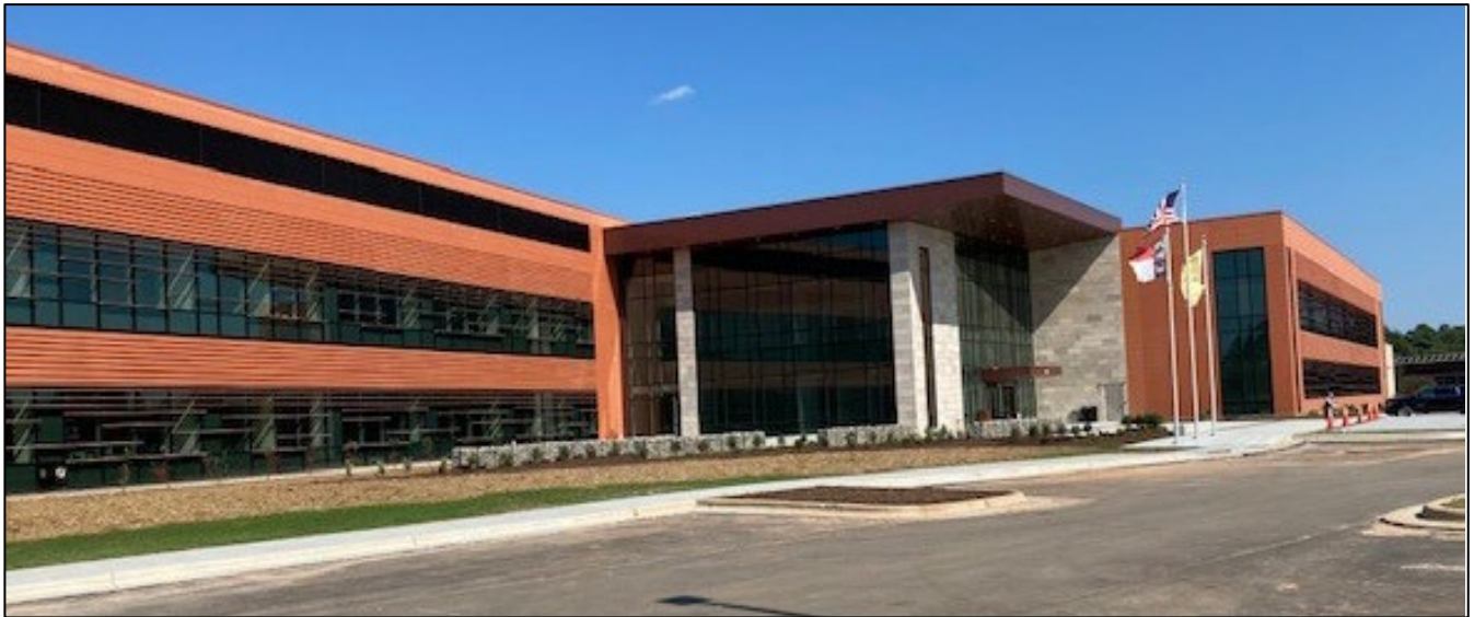
Agricultural Sciences Center, front view, with Main Lobby at center
